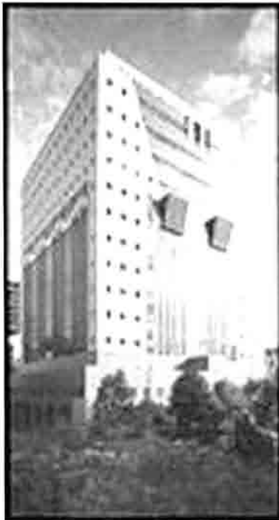
Municipal Service Building Portland, OR 1983
