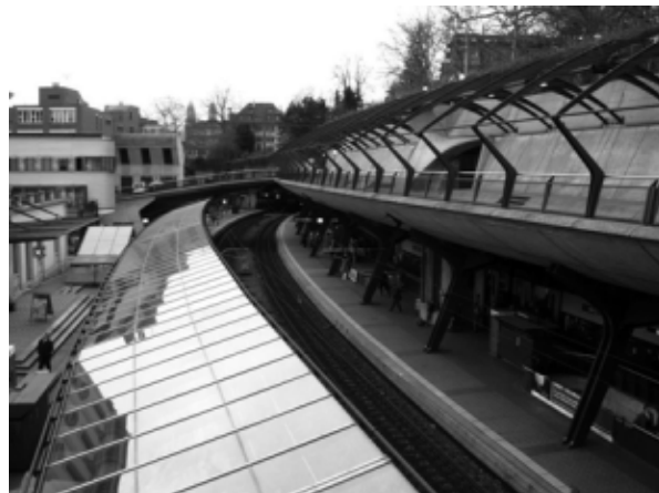
Stadelhofen Railway Station, Zürich, 1983–1990,
