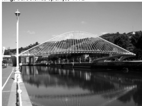
Campo Volantin Footbridge, Bilbao, Španija, 1994–1997,
