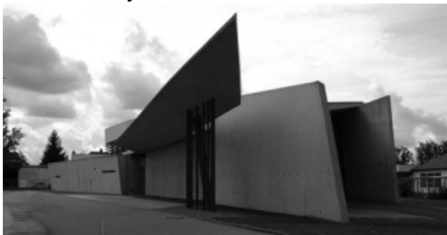
Vitra Fire Station, Weil am Rhein, Nemačka, 1990–94
