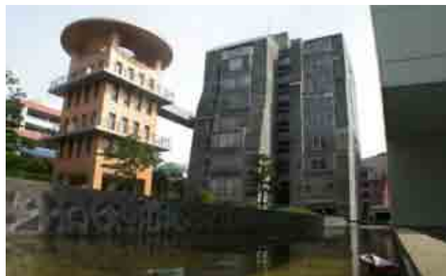
Stambena zgrada Nexus II, Fukuoka, Japan, 1989–92
